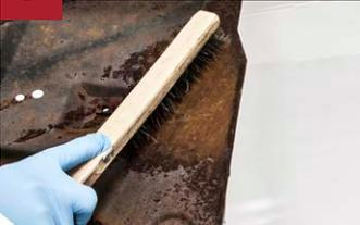
Remove loose scale with a wire brush. Clean with **SEM Solve** to remove oil, grease and dirt. Blow off with compressed air.
