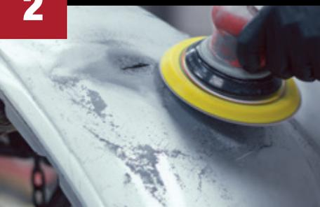
On front side, sand repair area with P80 grit. Dish out damage with P36 grit disc at a low RPM. On back side, grind repair area with P36 grit disc at a low RPM. Blow off surfaces. Re-clean if necessary.
